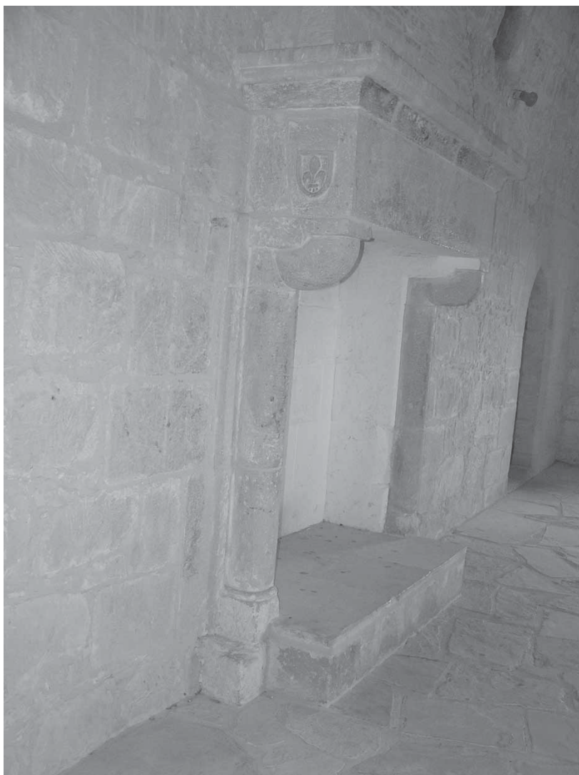
Fig. 84: Kolossi, keep, upper storey, southern room, fireplace [M. Olympios].
